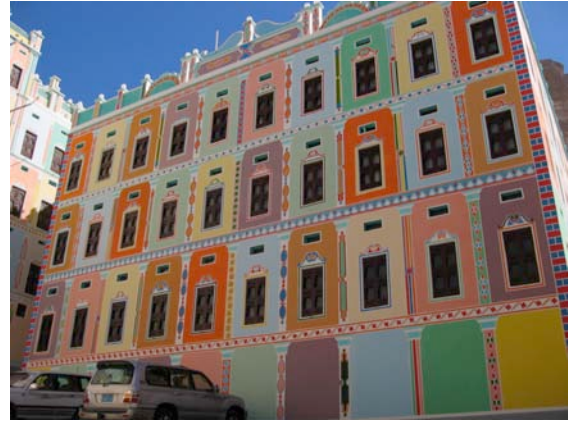
Fig. 49: New offices built next to the Bugshan hotel are constructed of mudbrick.
