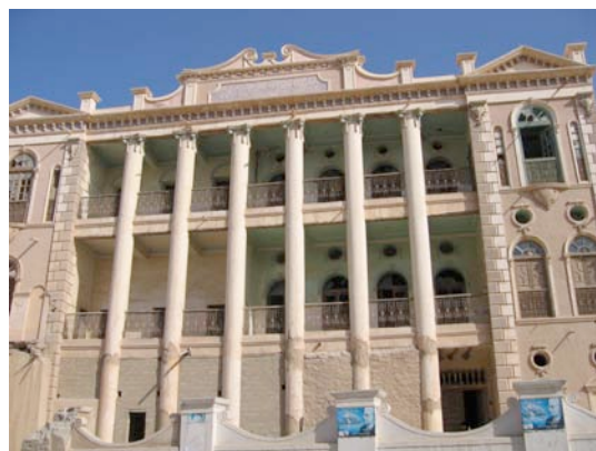
Fig. 17: Concrete block and mudbrick infill at the ground floor support buckling monumental columns in a temporary shoring measure.
